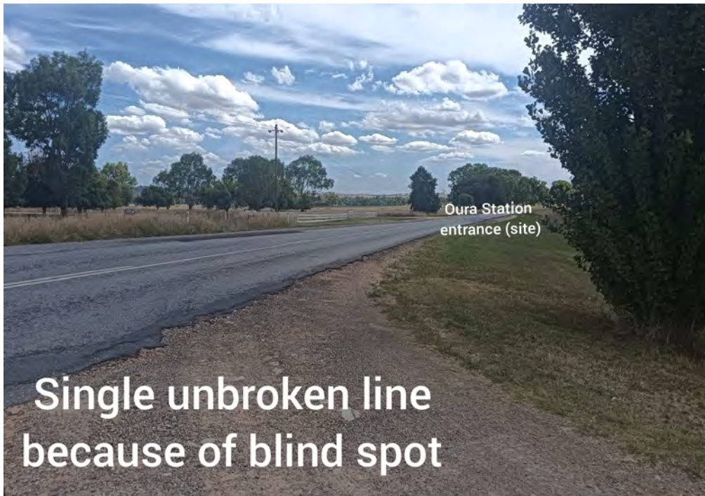
Figure 3. Unbroken single line on left of image due to blind spot. Oura Station (site) can be seen opposite with white rail fence.
