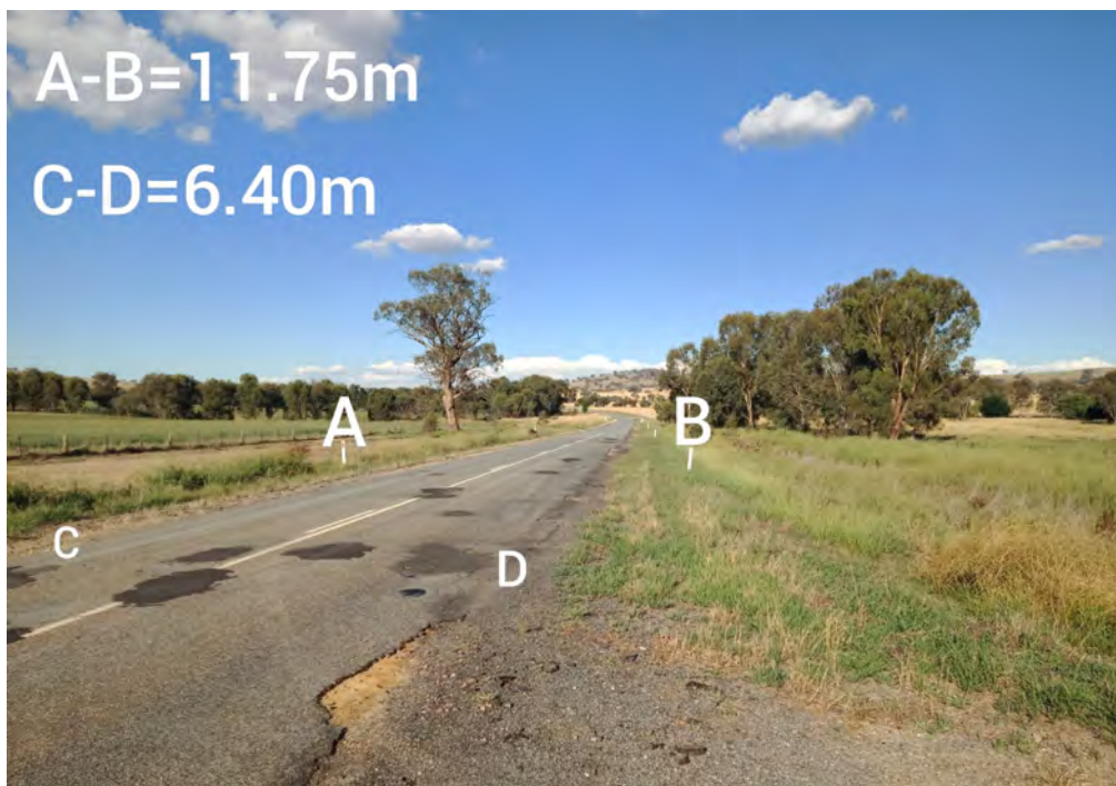
Figure 4. Road width shown east of Oura Station entrance, which is representative of the road both sides and at the entrance. Road width 6.4m
