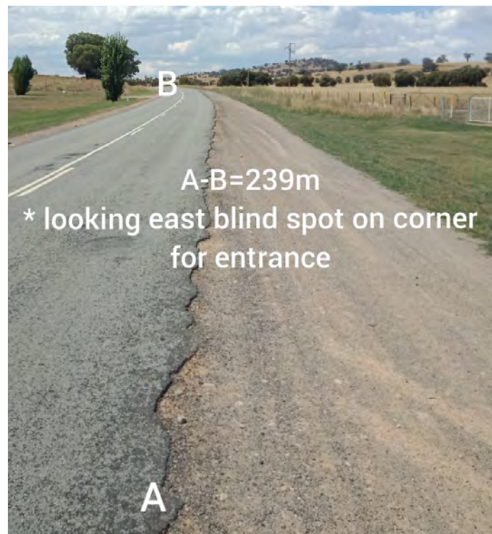
Figure 2. Oura road looking east, showing entrance to Oura Station on the right (point A) and the blindspot (point B), which effects vehicles travelling towards Wagga Wagga. This is also a school bus stop for morning pick-up (right side) & afternoon drop-off (left side) on the road.
