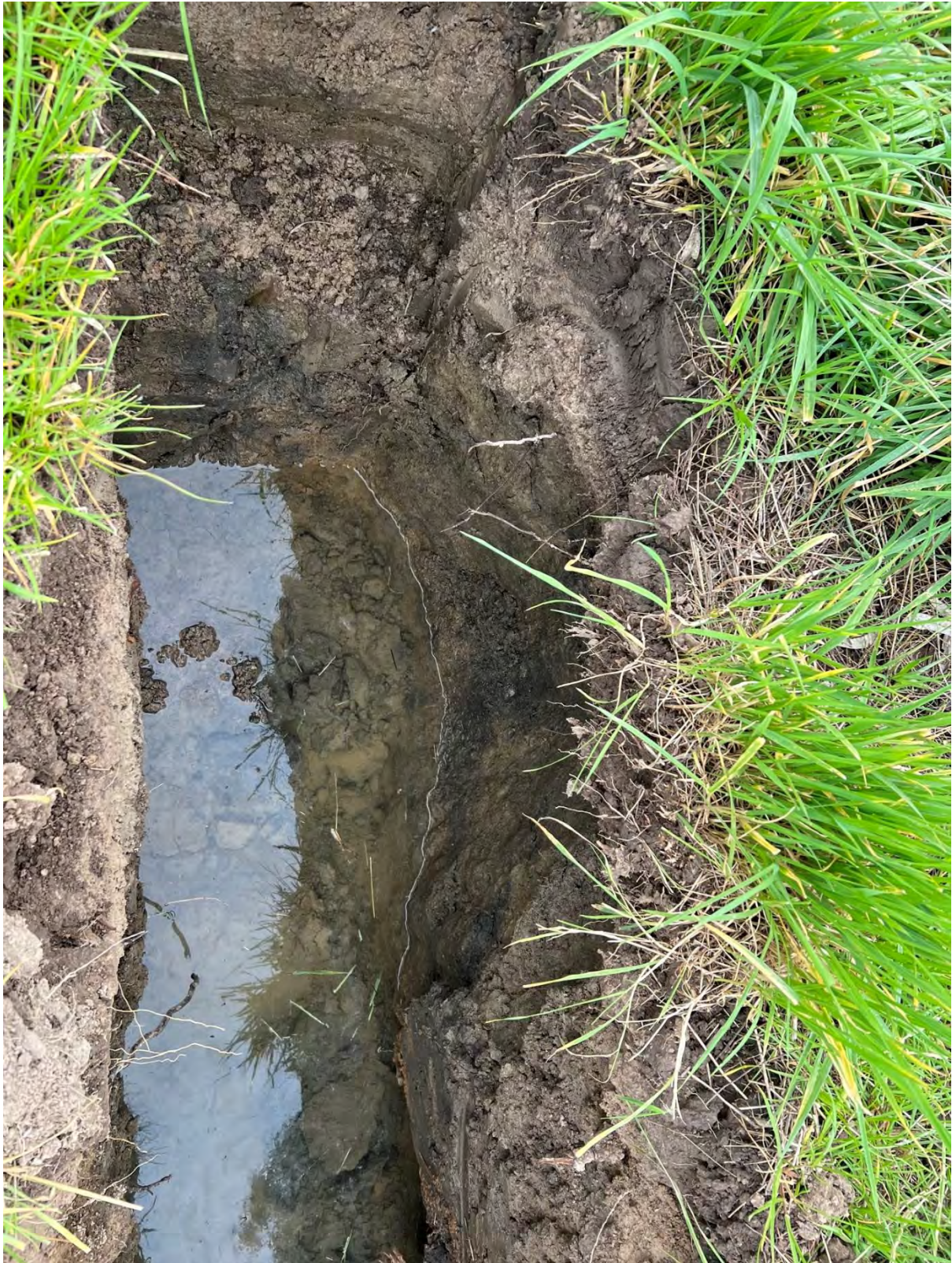
Photograph 2: Test pit 1 filling with water from interflow.
