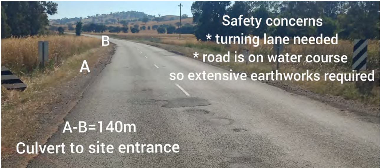
Figure 1. Oura Road looking east towards Wantabadgery showing watercourse, culvert (point A) and Oura Station entrance (point B). Distance is 140m.
